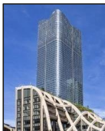
Azabudai Hills Mori JP Tower Completed: Jun. 2023
