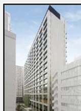
Omiya JP Building
