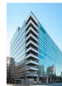
Kuramae JP Terrace (Constructed in March, 2023)
