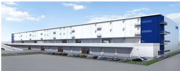
Aichi Post Office (Exterior)
