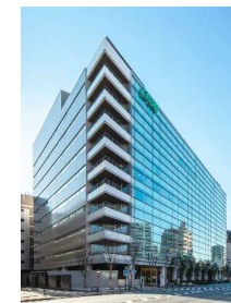
Kuramae JP Terrace (Constructed in March, 2023)
