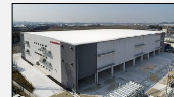
Logisite Kumiyama (Logistics facilities)
