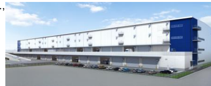
Aichi Post Office (Operations scheduled to begin in October,2025)
