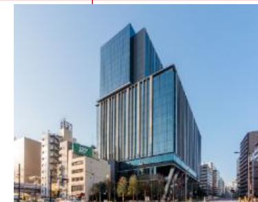
Gotanda JP Building
