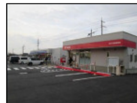
Saidaiji-Tomisaki Post Office (Okayama Prefecture) (Relocation on January 28, 2019)
