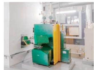
Boiler for thermal use of wood chips
