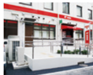
Ramp and handrails installed at the entrance
