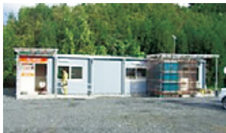
A temporary post office used by the Kamaishiheita Post Office (Iwate Prefecture)
