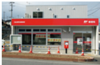
Reconstructed Ofunatoekimae Post Office (Iwate Prefecture)
