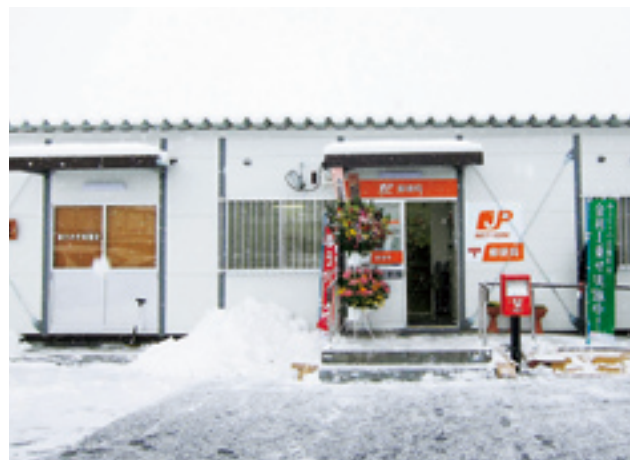
A makeshift office used by the Arahama Post Office (Miyagi Prefecture)
