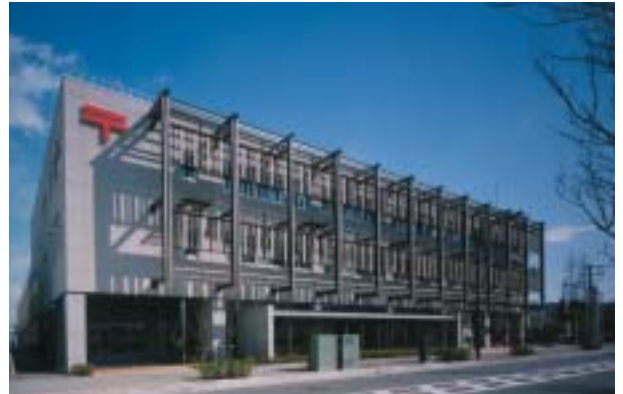
Odawara-Higashi Post Office External view
